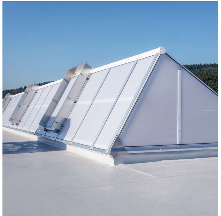
LAMILUX Continuous Rooflight S a Kemper GmbH olpei ipari csarnokán
