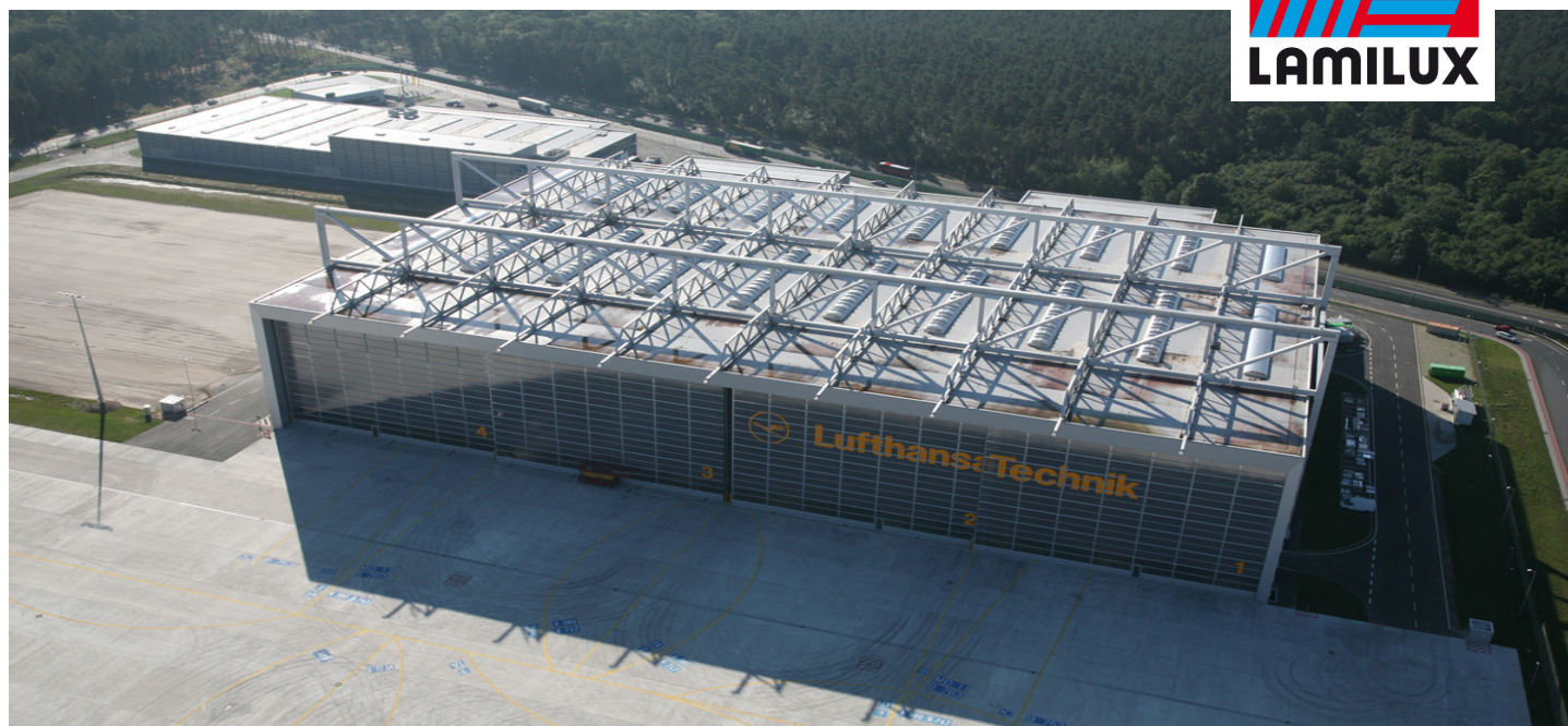
A380 Assembly Hangar
